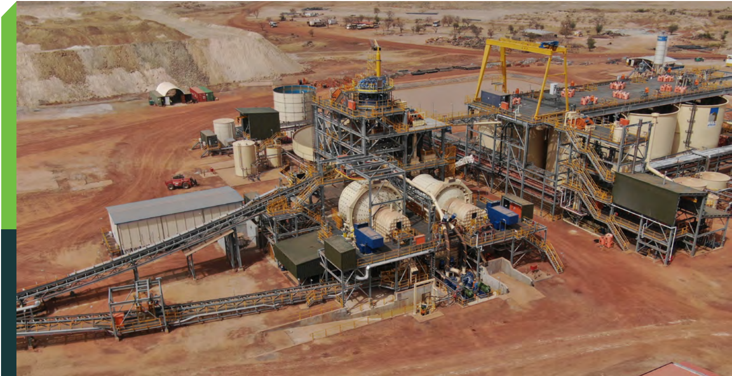
Sanbrado Gold Mine, Burkina Faso
