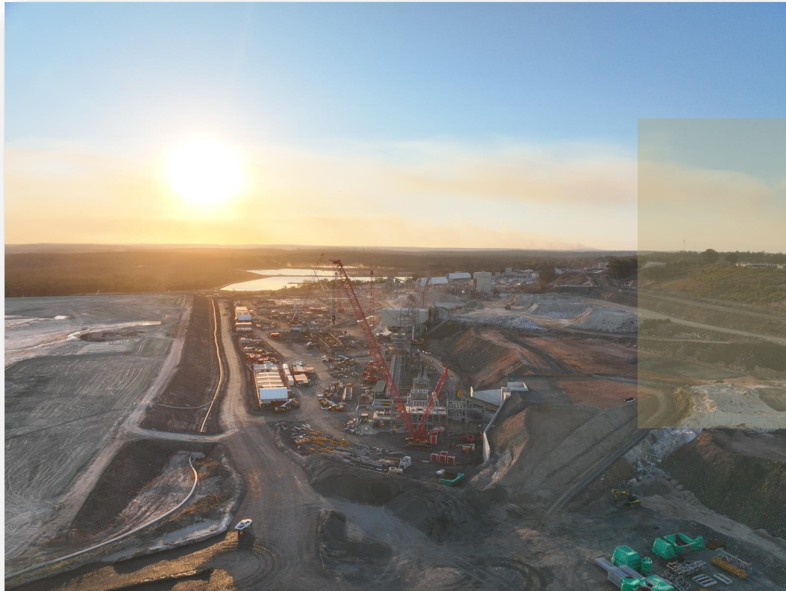
Chemical Grade Processing Plant #3 Project, Western Australia
